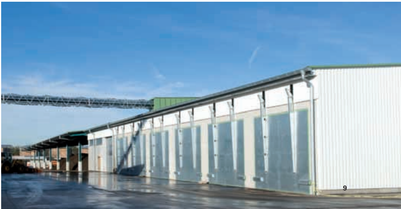
The core of the plant: the garage-like digesters
